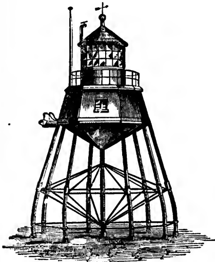
The Maplin Lighthouse, erected by Mr. Walker, upon Mitchell's screw-pile foundation.
